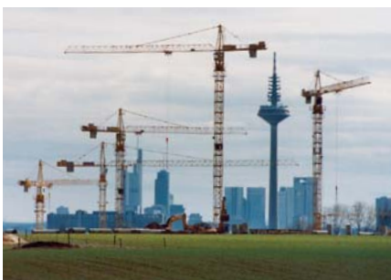
Summer 2002, first signs of construction
